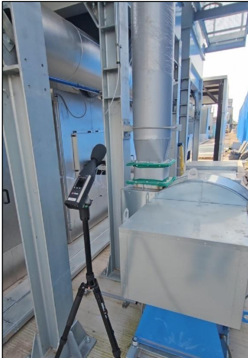
Fig 8b – Regenerative Thermal Oxidiser (RTO) Burner Motor (2) & Outlet Pipe (3)
